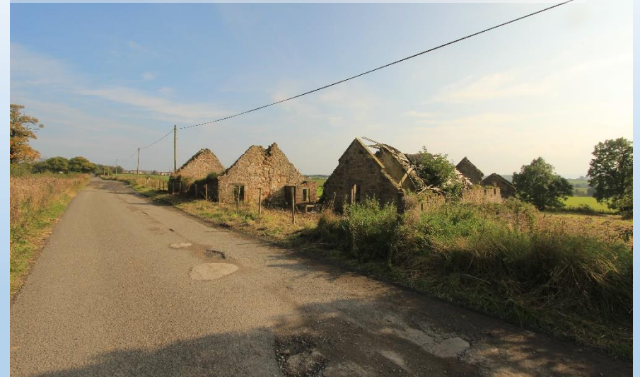
The private tarred access road is on the left of the ruin
