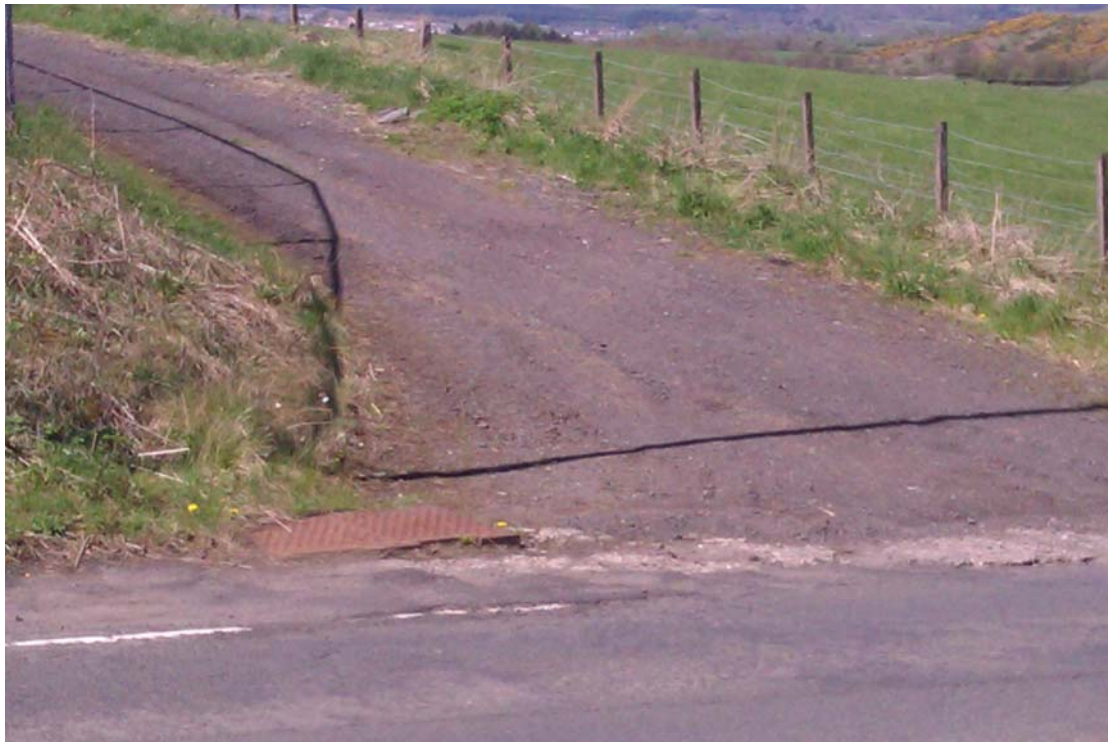
Adjacent access to housing site
