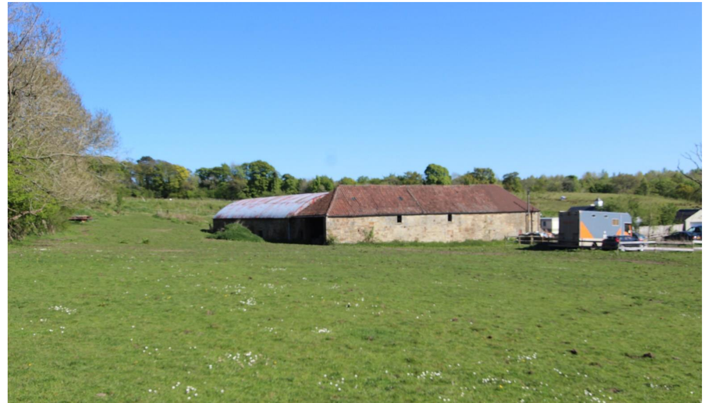
Picture shows the paddock and the western elevation of the barn. Front page picture shows the western elevation
